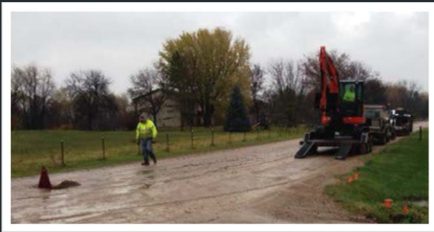
Repairing a collapsed drain tile in the rain
