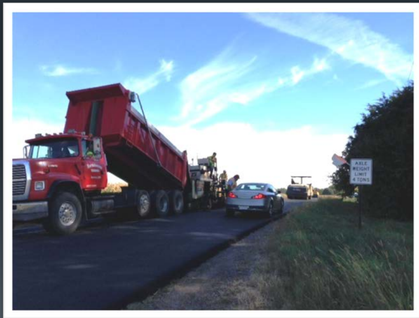
A 14 hour day to complete the blacktopping
